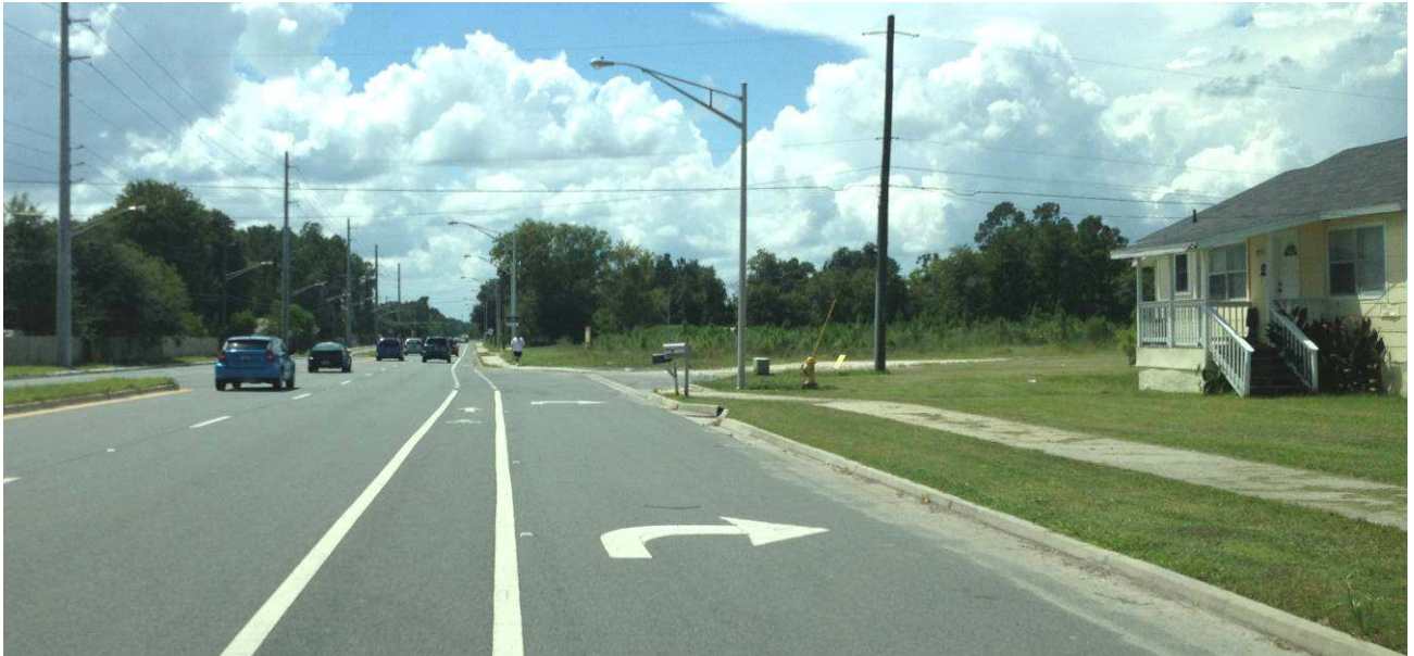
Subject site on the right facing west along Collins Road
